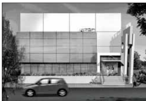
Newly constructed building for AEPC-Knitwear Technology Mission in Tirupur
